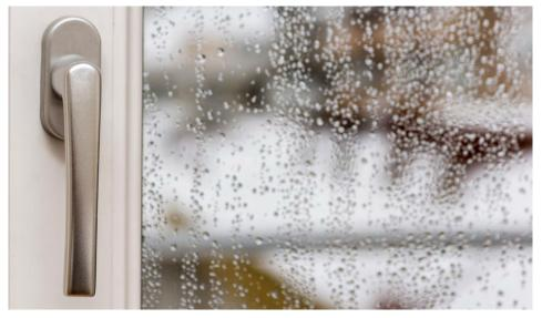
Moisture condenses when cold surfaces meet warm moist air. Condensation will make surfaces wet, which can cause water damage or help mould/mildew grow.
